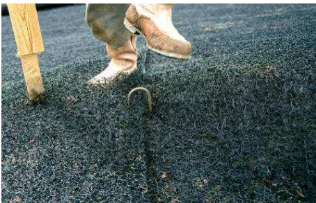
Typical U-shaped mild steel fixing pins
